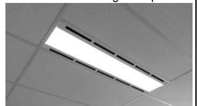
T-Bar mounting example
