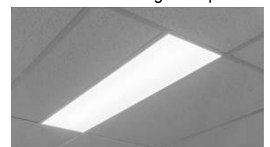
T-Bar mounting example
