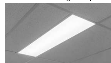
T-Bar mounting example
